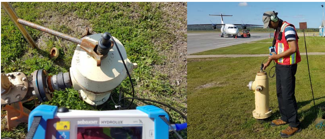
Figure 1. Hydrant sounding at an airport
