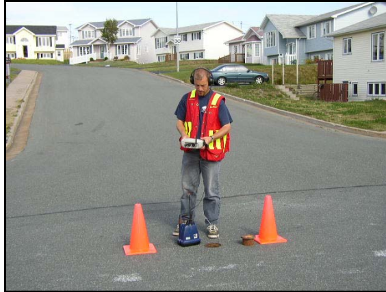
Correlating a leak from a valve
